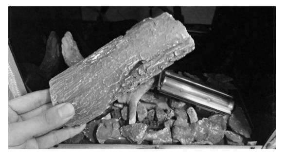
Place log A on the burner tray base at the back of the fire as shown in this picture.
